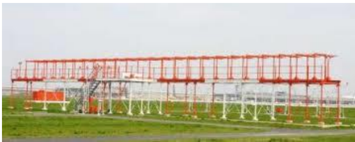
Figure 2.2c ILS Localizer Antenna Array
